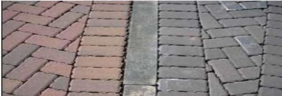
Superficies Permeables (Permeable Paving)
